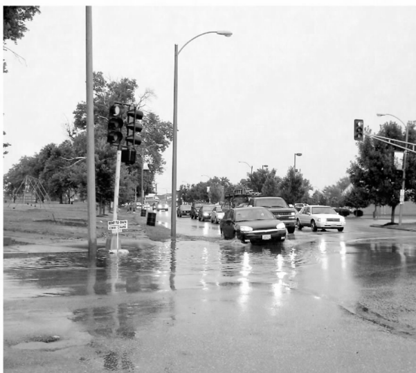
Standing water stretches more than 100 feet along Broadway at Meramec Street during Wednesday night's storm. Traffic backed up, and pedestrians trying to cross the street got soaked in water that, in places, was more than a foot deep. The Metropolitan Sewer District says that it is working on the problem but that it won't be fixed until next year. Matthew Hathaway
